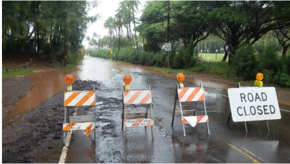
South Kihei Road flooding April 2017
