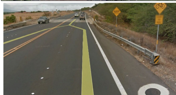
Pinch location at Keokea Gulch Bridge on Piilani Highway south bound (Source: Google Maps)
