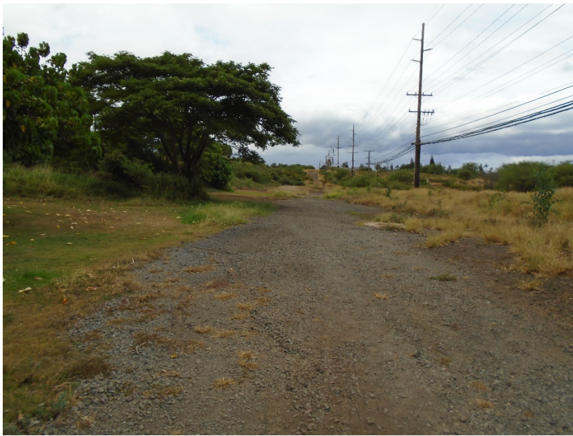
Future North-South Road Phase 3, south of Halekuai Street
