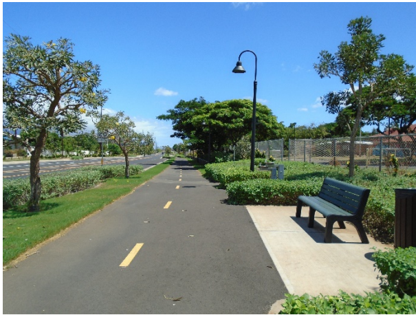
Completed section of Kihei Greenway, fronting Lokelani Intermediate School
